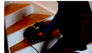
Cleaning of inside stairs
